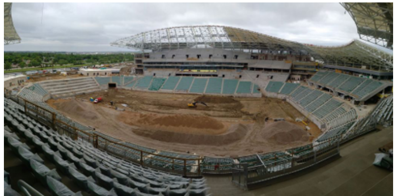
The new Mosaic Stadium during construction.
