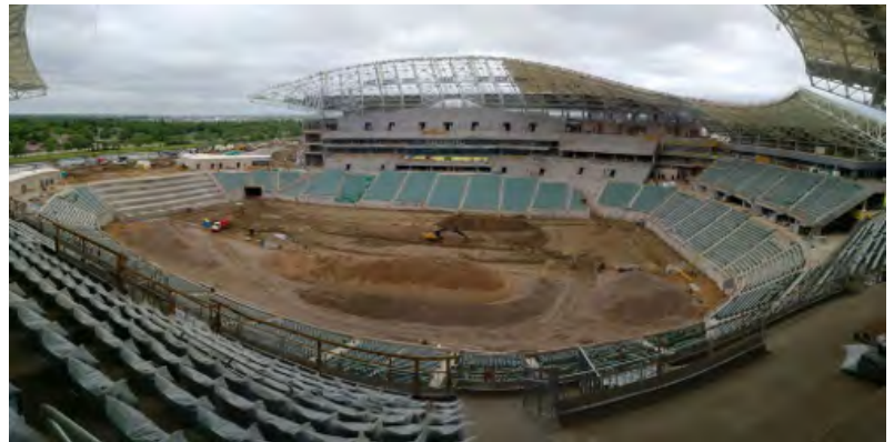
The new Mosaic Stadium during construction.
